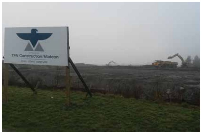
Chevron cardlock fueling facility site preparation works completed January 2015
